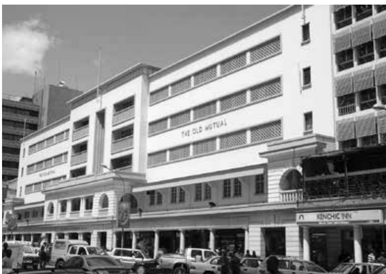
The Old Mutual. The insurance company fears that gazettement will block redevelopment and lower its value. Photo by Akbar Hussein.
