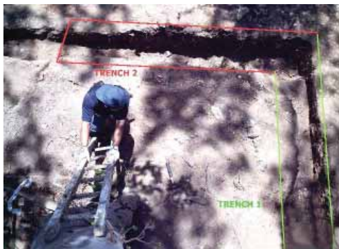
Top view of trenches 1 and 2.
