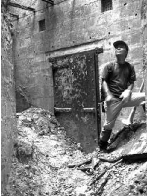
Surveyor T. Yokogawa inside one of the three underground operation rooms found in the cliffs below Bandari College, overlooking Kilindini Harbour, before they were sealed off in 2008. Photo: Hans-Martin Sommer.
