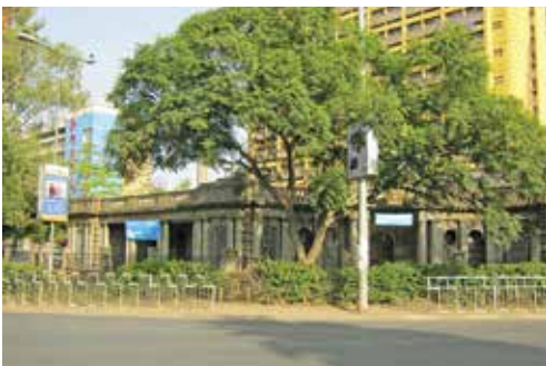
The first Provincial Commissioner's house was designed by architect C. Rand Overy.
