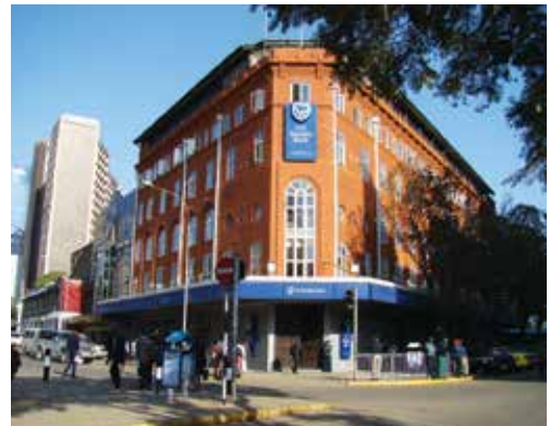
Stanbic House was designed by architects Henderson and Partners, who also built the Muthaiga Club.
