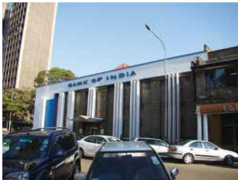
Under the Bank of India façade lies the original stonework of the Memorial Hall building.
