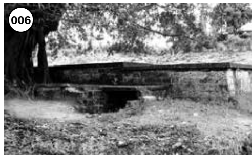
Entrance to the underground generator bunker.
