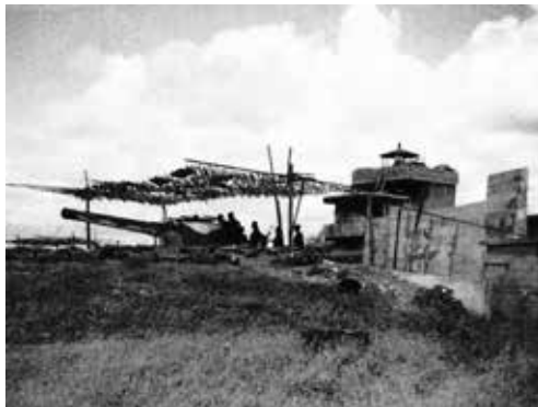
Training of gunners on the No. 2 battery in 1936/37. In the background can be seen the Battery Observation Post with the umbrella-protected rangefinder on top. Photo: The National Archives, Kew.
